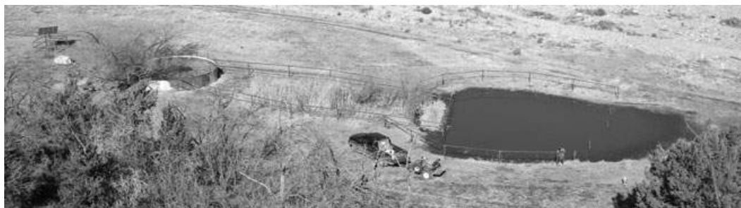
Fig. 1. Windmill- and solar-powered pump installed to retain water levels in ponds (Turner Ranch Properties, L.P.; M. Christman, US Fish and Wildlife Service, Albuquerque, NM; photograph: C. Kruse, Turner Enterprises, Inc.; pers. comm.).
